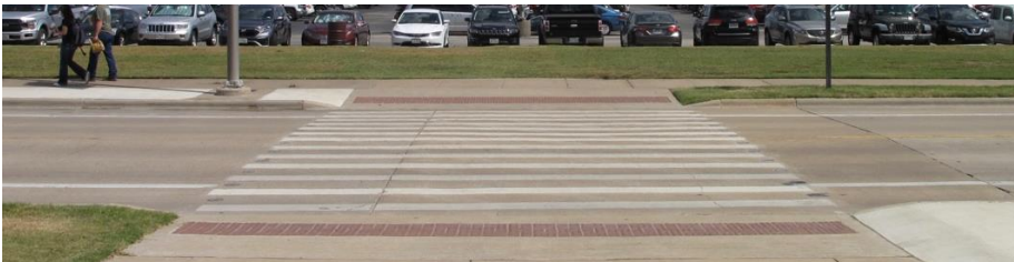
Figure 92: Walkway at PEAP across Penberthy Boulevard
