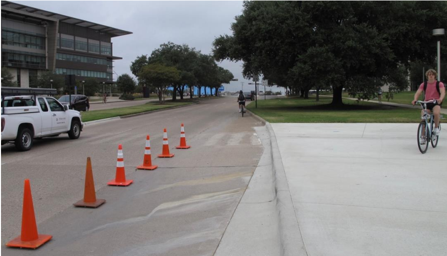
Figure 132: Cones demarcate the bike lane, which ends north of Polo
