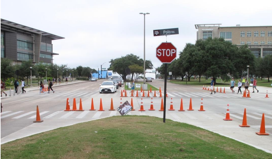
Figure 129: Cones creating pedestrian refuge in median of Bizzell Street
