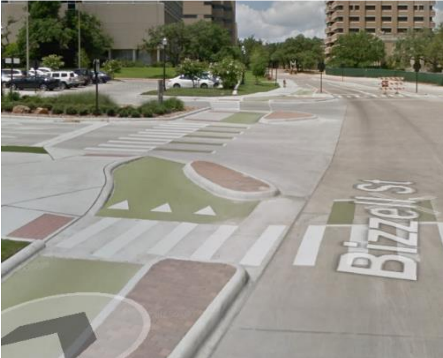
A portion of the “Dutch-style” intersection at Bizzell and Ross Streets on campus. Source: Google Maps.
